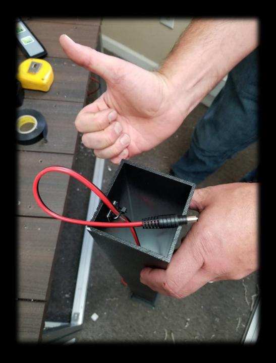
TIP: Install an adhesive anchor and zip tie to hold the wire at the top of the post.
