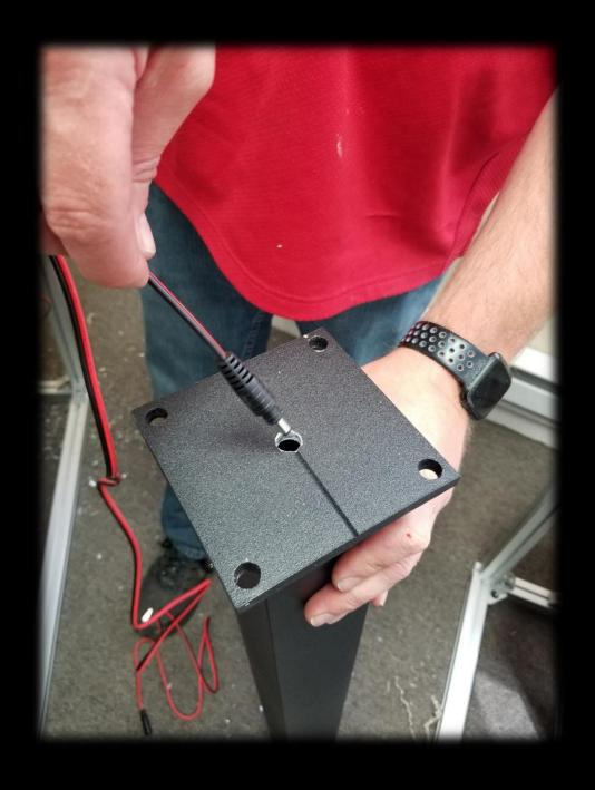
Feed the male end of the harness into the hole at the bottom of the post.
