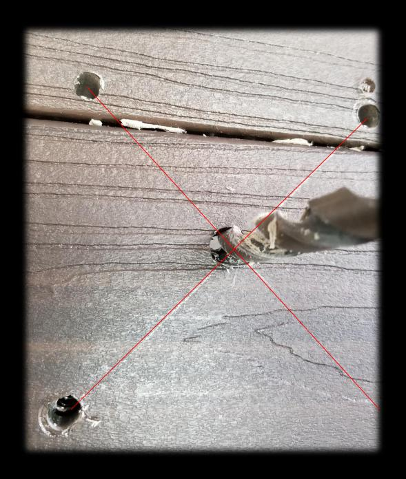
Mark the center point where the post will mount, and drill a ½" hole in the deck surface.
