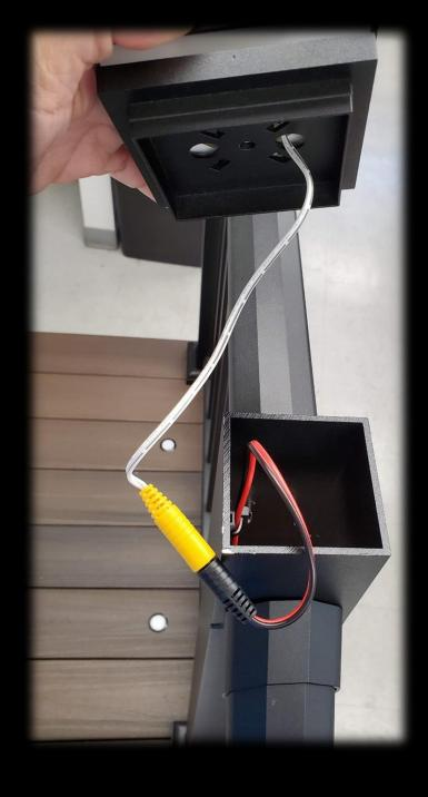
Plug the cap light into the male connector at the top of the post.
