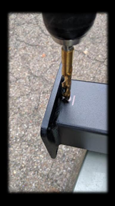
Drill a ½" hole in the base of the post closest to the transformer, this will be the only post needed drilled as such.
