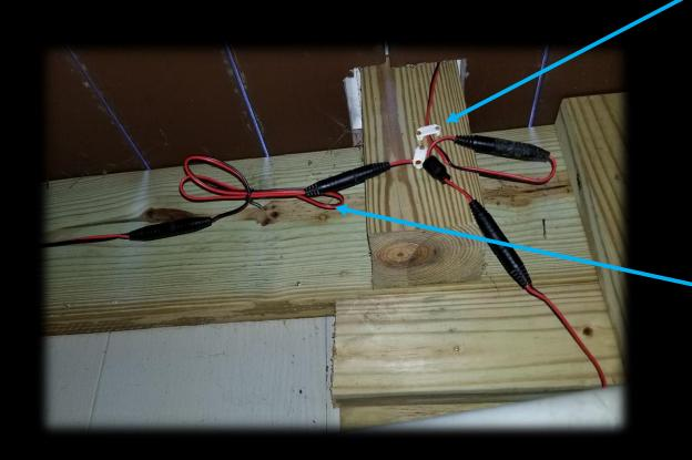
Secure the harnesses below the deck with insulated wire staples as shown.
