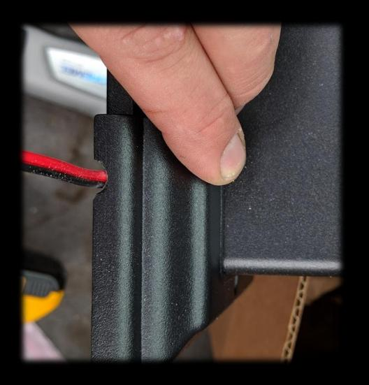
Notch the bottom of the skirt to allow the wire to pass through, while staying flush with the deck.
