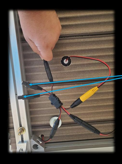
Place caps (provided with 5 output splitter) on any of the unused outputs to prevent corrosion and shorts.
