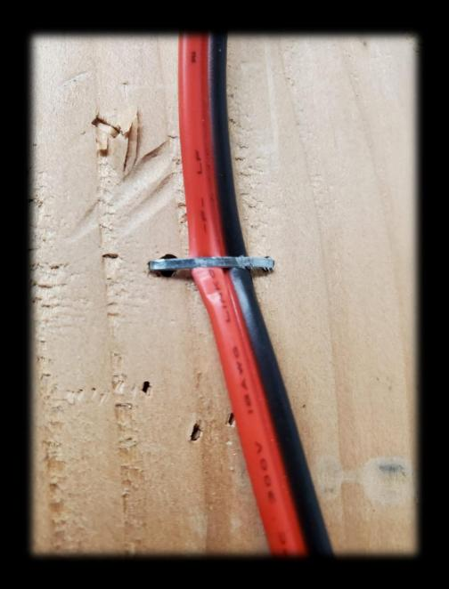
DO NOT use uninsulated wire staples, like pictured. If installed too tight, staples will cause damage to the wire.
