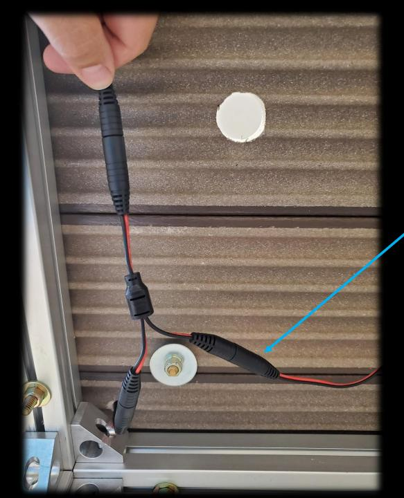
The remaining output from the splitter is then used to continue the main harness to the rest of the system, running directly to the next post.
