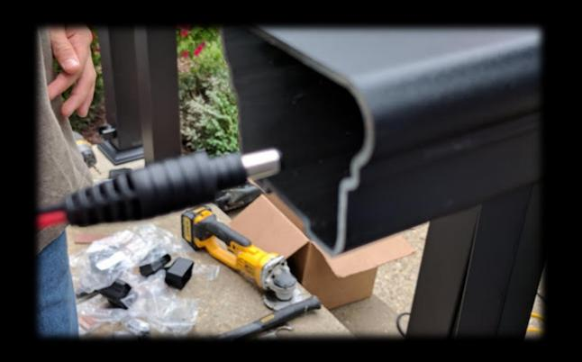
Upon drilling a hole in the post, insert the harness into the rail.
