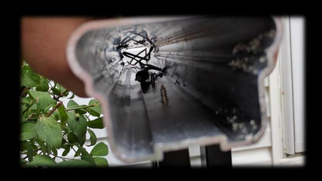
Run the wire through the hole drilled in the post, then through the top rail. Drill a hole in the receiving side of the next post, and repeat the previous process.
