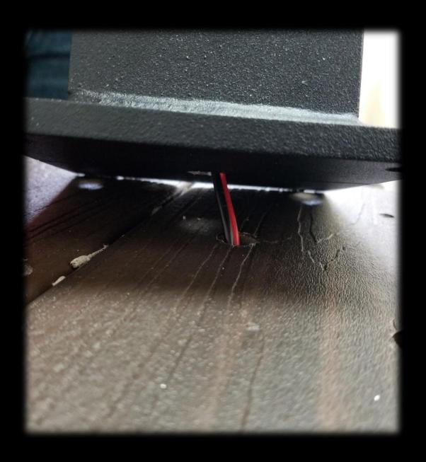
Make sure the wire moves freely into the hole and does not get pinched under the post.
