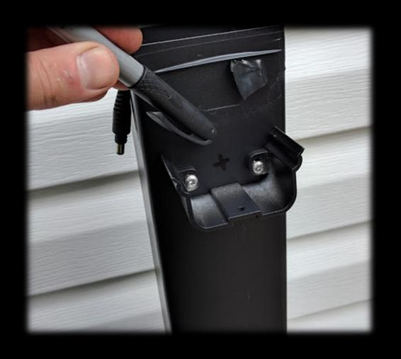
Run the harness up the post and hold it at the top of the post using electrical tape. Screw in the top rail bracket. Mark the post and drill a ½" hole for the connector to go through.
