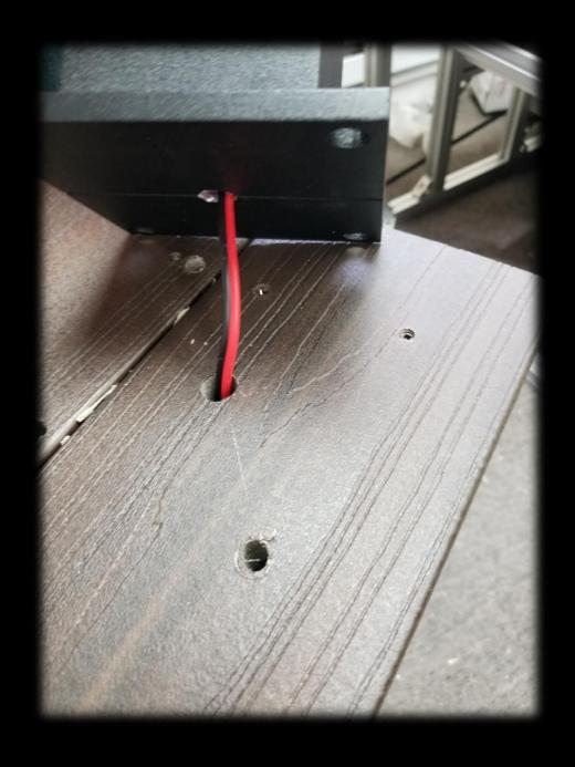
Continue to feed the harness as the post is placed into position on the deck.
