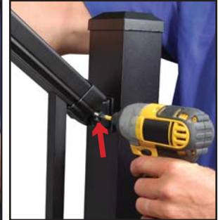
(b) Anchor Bracket w/ pivot screw
