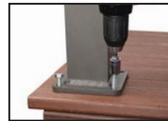
Fasten Post to Deck Surface
