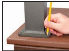
Mark and Pre-drill Holes
