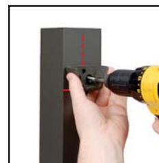
Center bracket and attach to post
