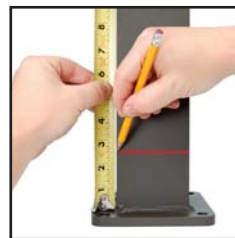
Measure up 2-1/2" from top of base plate
