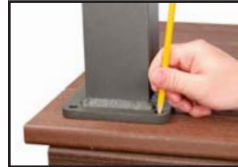
Mark and Pre-drill Holes
