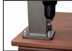
Fasten Post to Deck Surface
